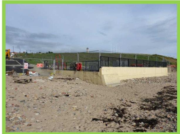
Yellow painted sea wall at site of former Boardwalk Cafe (/4501C09)
