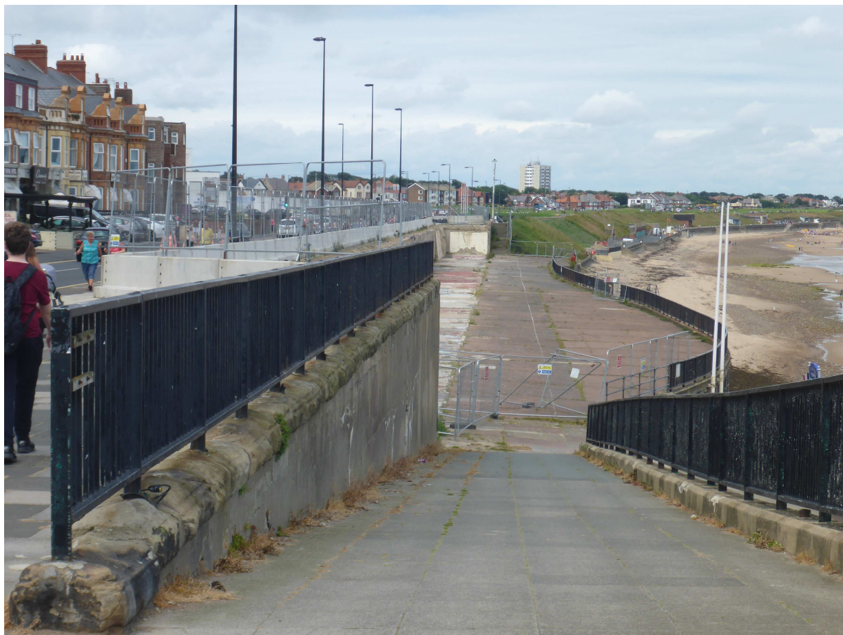
Area of Whitley Bay lower promenade closed-off awaiting redevelopment as part of Seafront Master Plan
