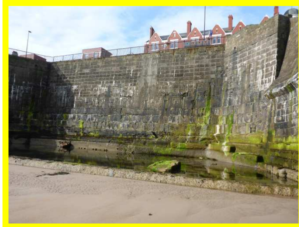
High blockwork sea wall (/4601C05)
