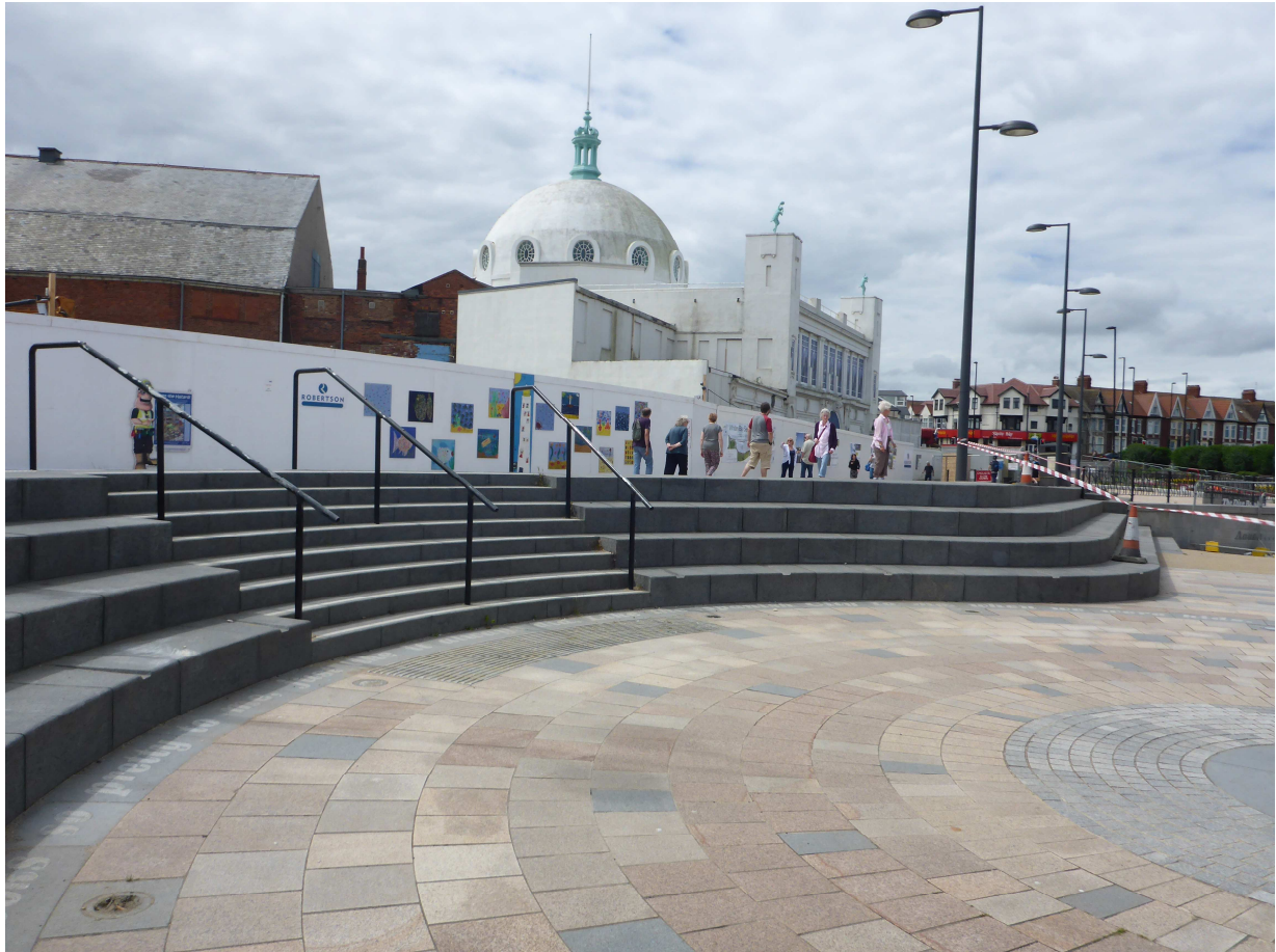
Area of Whitley Bay upper promenade near Spanish City already redeveloped as part of Seafront Master Plan
