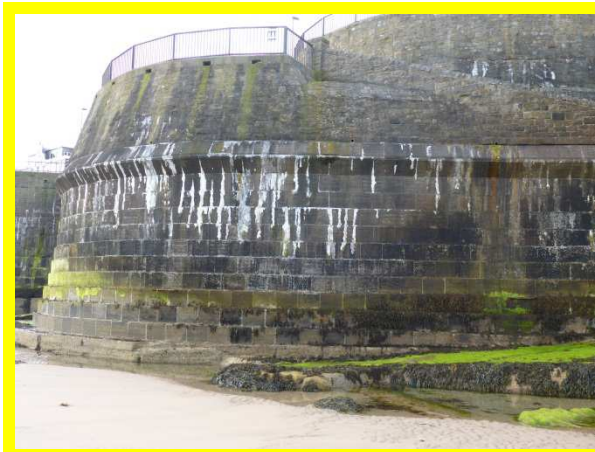
Blockwork sea wall at first 'bullnose' (/4601C04)
