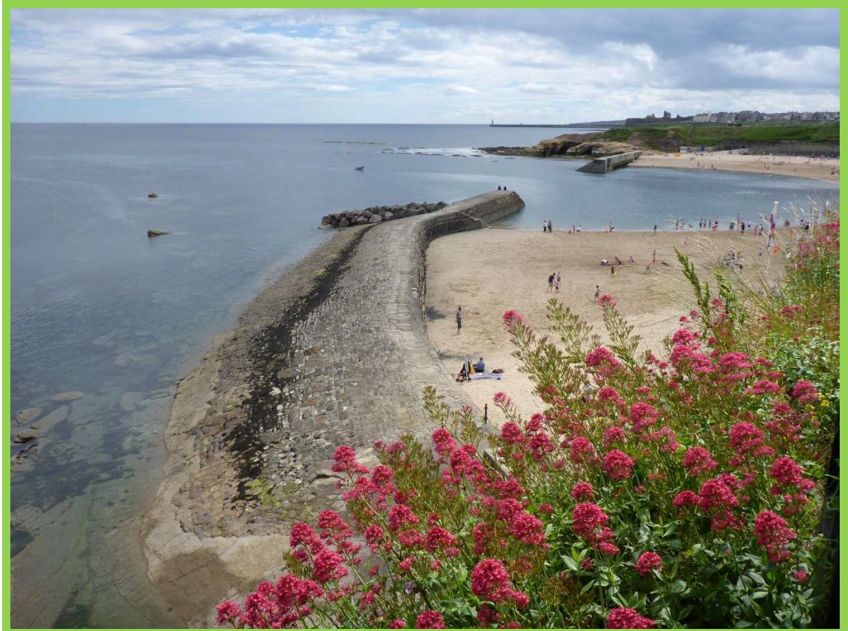
Cullercoats North Pier in good condition following repair works (J4701C07)
