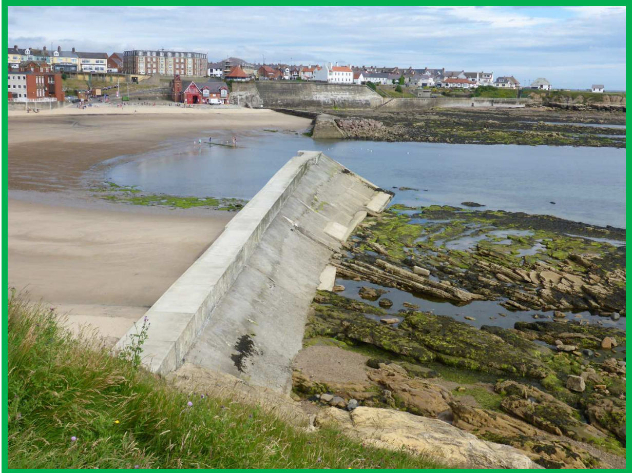
Cullercoats South Pier in very good condition following refurbishment works (I4701C15)
