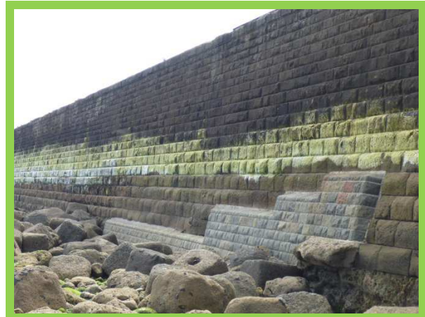
North Pier appears in good overall condition and is well maintained (/4801C01) Areas of previous repairs at toe (/4801C01)
