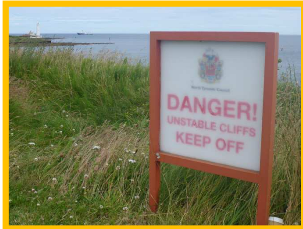
Warning signs along cliff top at municipal golf course (/4501C05)
