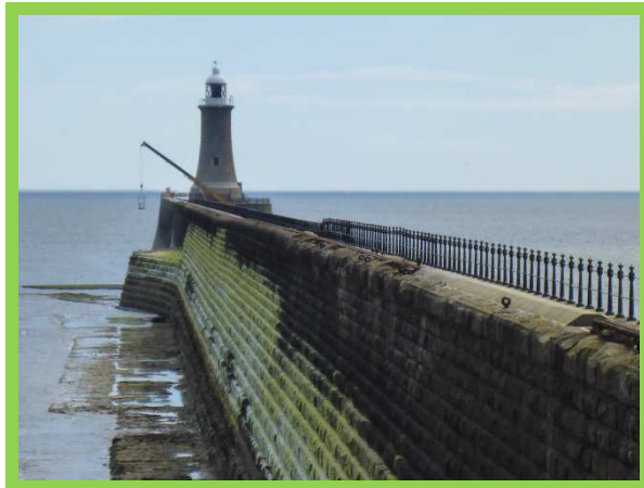
North Pier appears in good overall condition and is well maintained (/4801C01) Areas of previous repairs at toe (/4801C01)
