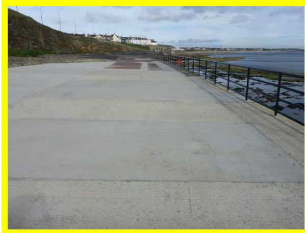
Repaired deck following storm damage in 2013 (/4601C08)
