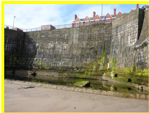
Blockwork sea wall at second 'bullnose' (/4601C06)
